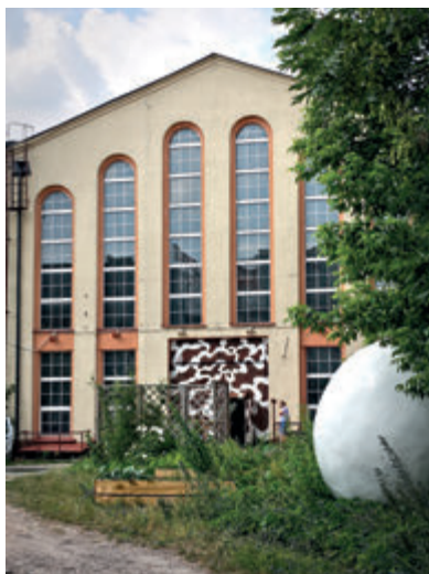
The building of the former power plant, photo by I. Czajkowska
